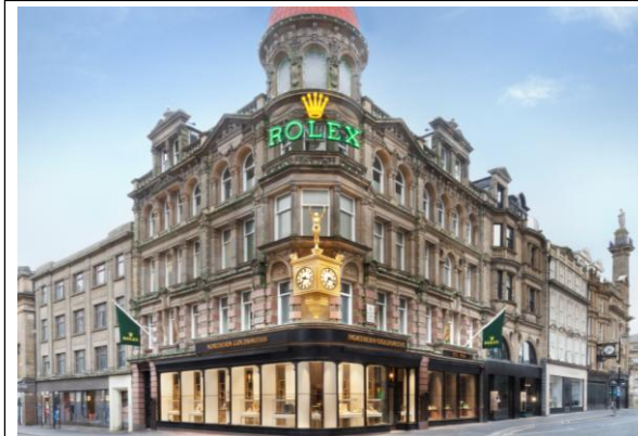
Northern Goldsmiths Newcastle Refurbishment Jul 25
